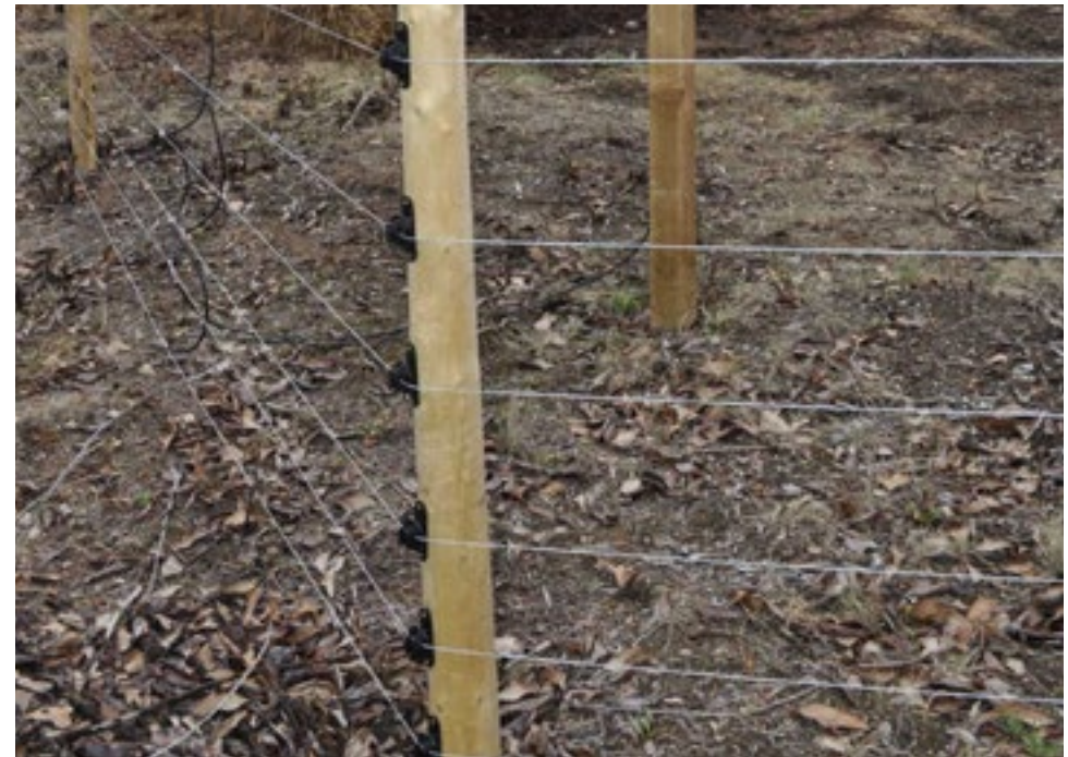
Post and insulators
